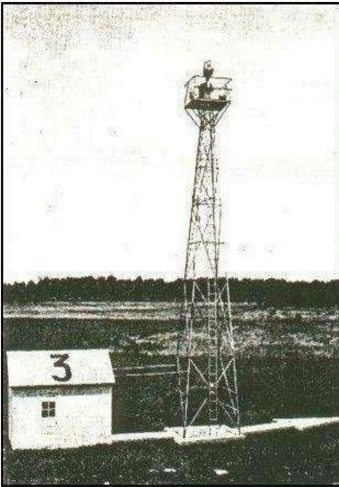
Beacon site at intermediate landing field, Cleveland–Albany route. The "3" on shed roof signifies beacon 3 of 10 in this sector.
